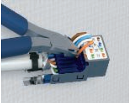
Device connection – shorted cable excess Cut off the excess cable length with cutters.
