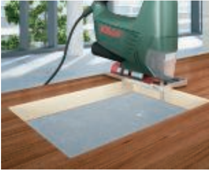
Preparation for Deskbox mounting A rectangular mounting opening is required for Deskbox installation. The appropriate installation dimensions can be found in the mounting instructions.
