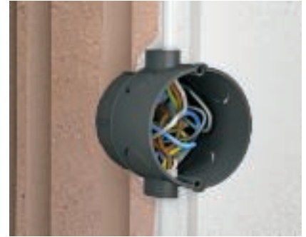
Device connection sockets Device connection sockets have a total compartment volume for the installation of an installation device and also space for at least three connection terminals.
