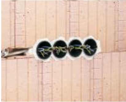
Accessory mounting box installation Concealed devices and connection sockets can easily be plastered into masonry of all kind.
